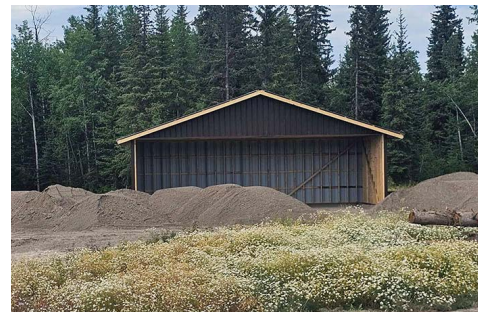
New builds progressing: Wood shed.
